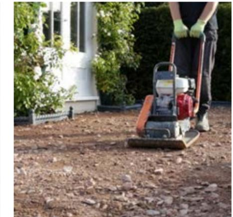
2. Prepare the ground as normal with compacted hardcore, achieving the correct falls for drainage.
